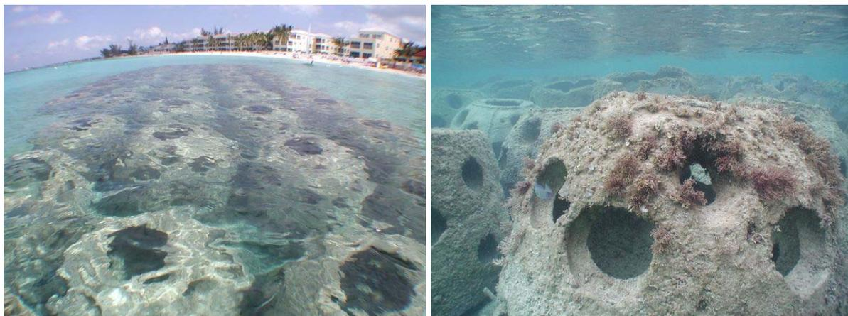
**Figure 6. Photographs of 5-Row Reef Ball Breakwater offshore Grand Cayman**
