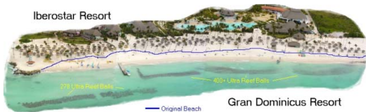
Figure 2. Aerial Photograph of Dominican Republic Projects
