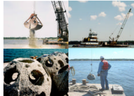
Mill Hill Oyster Sanctuary Installation & Field Test
